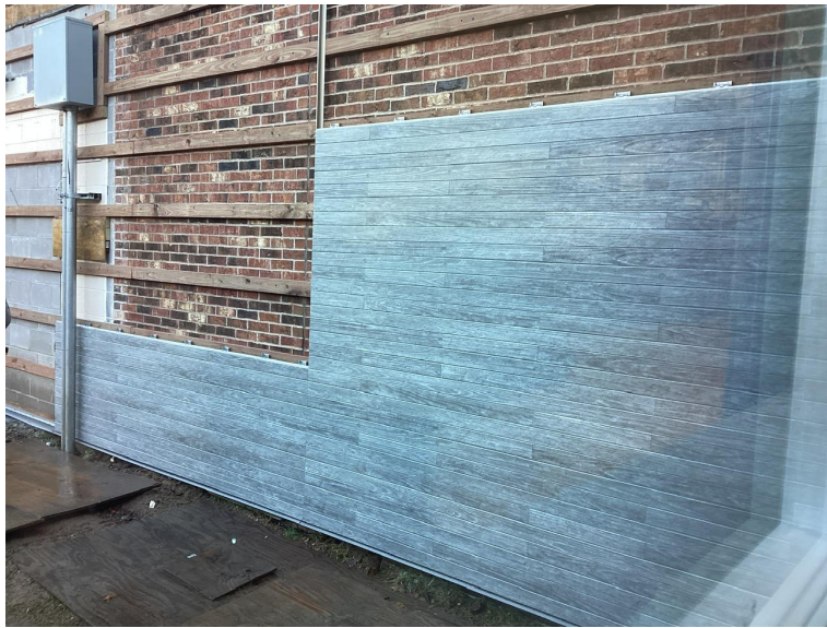
Ceraclad Wall Finish in the Cafeteria Courtyard
