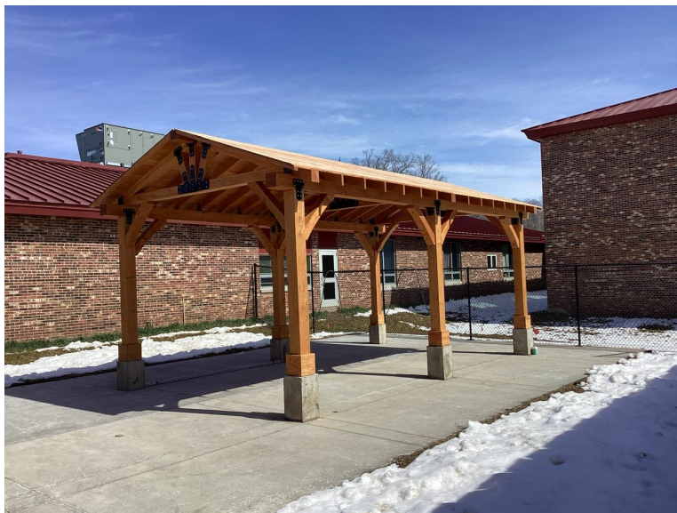
Cafeteria Courtyard Pavilion Installed
