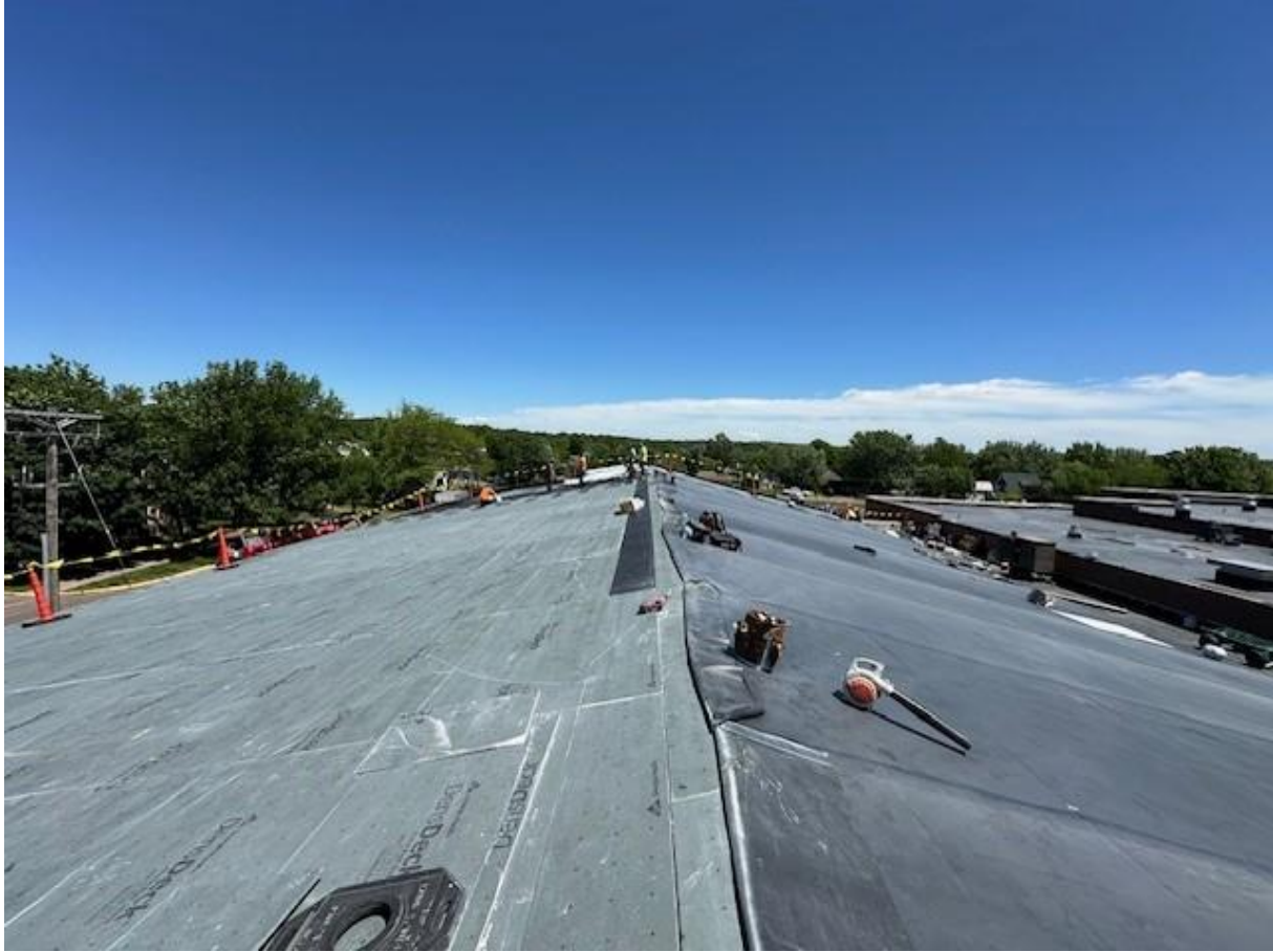
Re-roofing of Elementary School (Gym is only area remaining)
