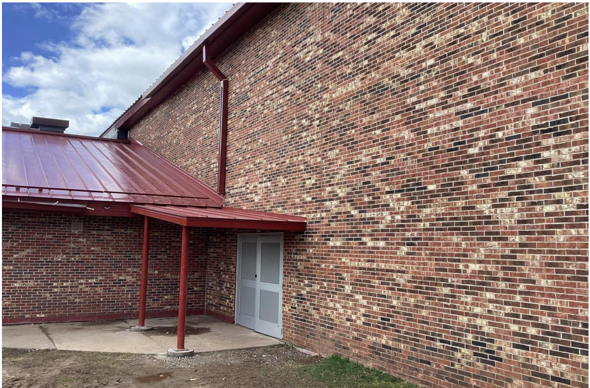
Brick Washing Completed and Canopy Over Exterior Door Installed
