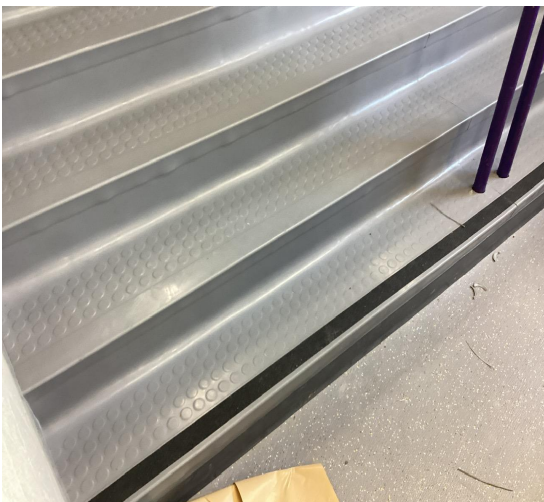
Stair Tread Flooring Finishes Installed
