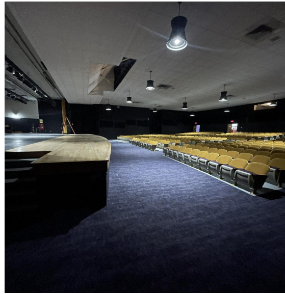
Auditorium Ceiling Completed
