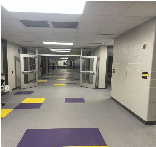
Installed Magnetic Hold-opens on Security Doors
