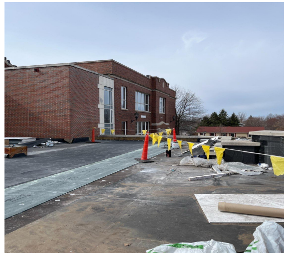
Roofing Work at Ladysmith Elementary
