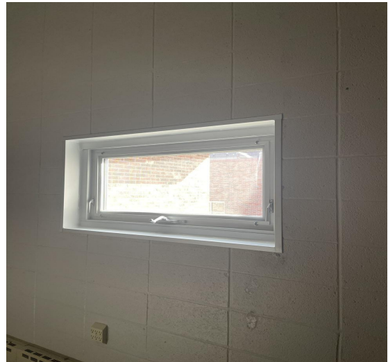
New window installed at Room 410 - Conference
