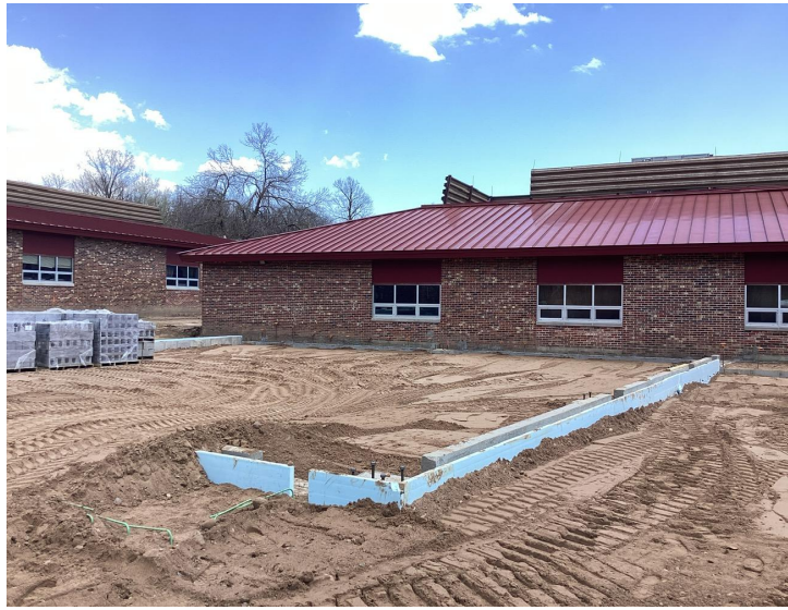
Media Center Foundation Walls Backfilled/Compacted
