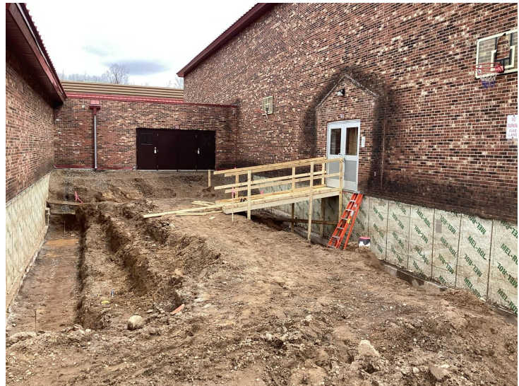
Excavation at New Corridor
