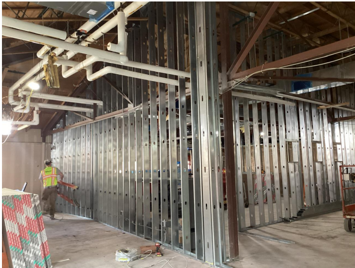
Framing at Existing Library/Media Center
