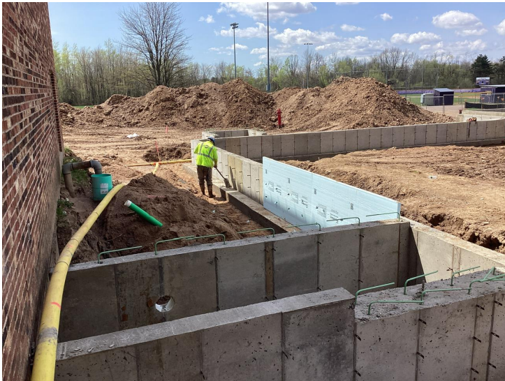
New Gym Foundation Walls Poured
