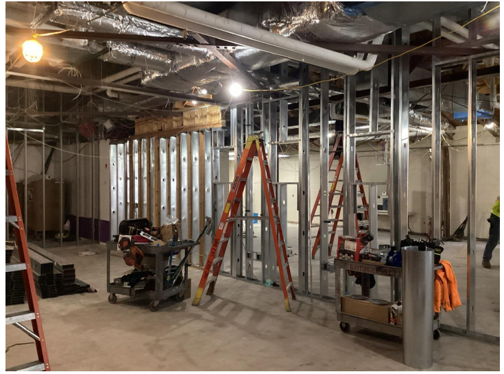
Electrical and Mechanical Rough-ins at Existing Library
