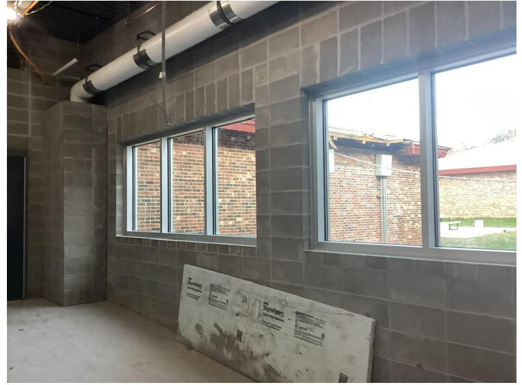
Building envelope dried-in at Gym addition corridor
