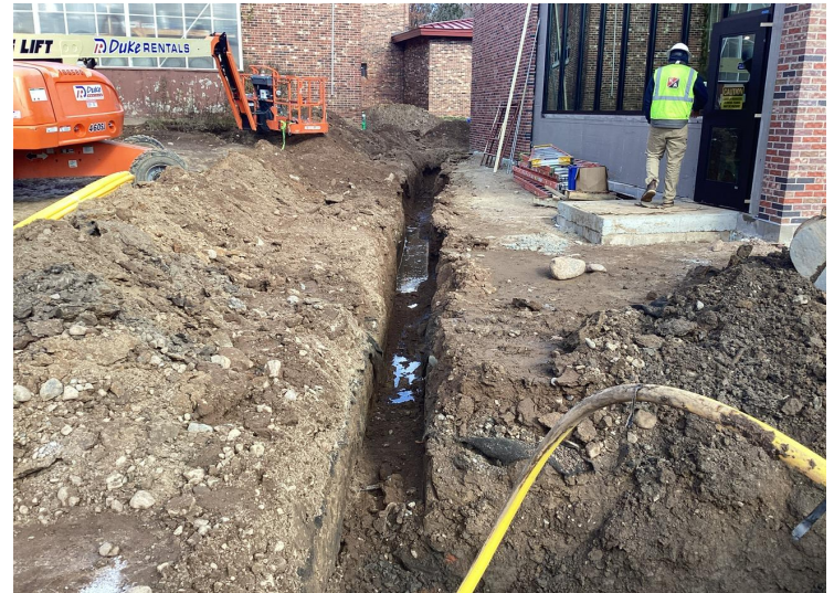
Gas line being trenched to serve new generator
