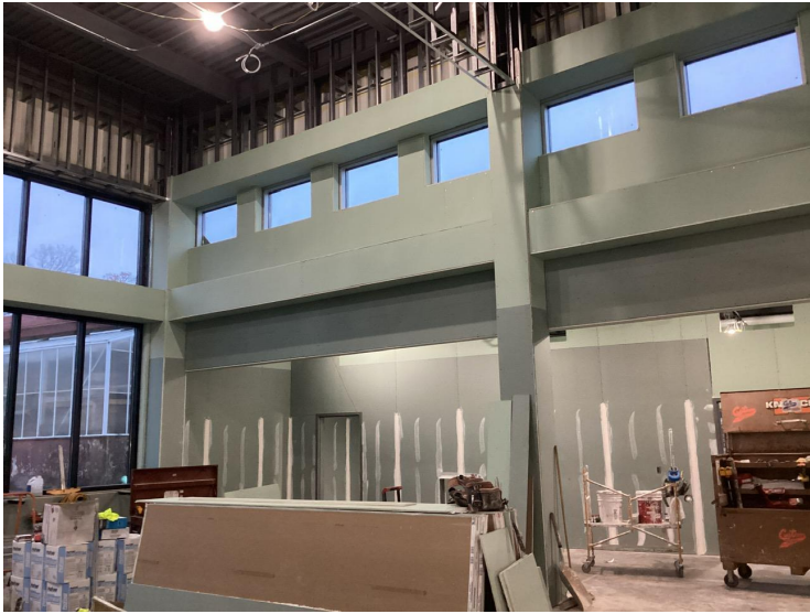
Drywall being installed at Media Center addition
