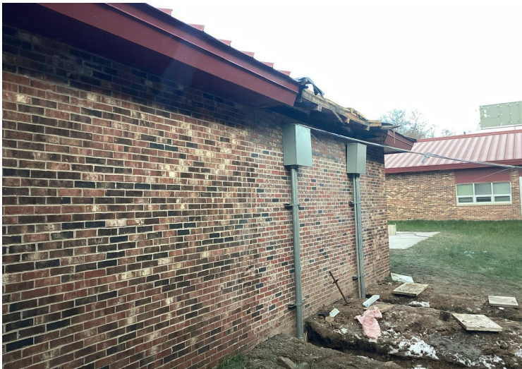
Existing electrical lines trenched from existing gym to cafeteria
