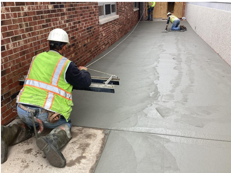
Concrete flatwork being completed at Gym addition
