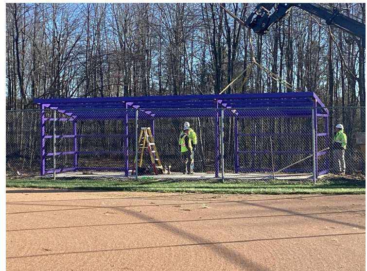
Softball dugouts are being installed
