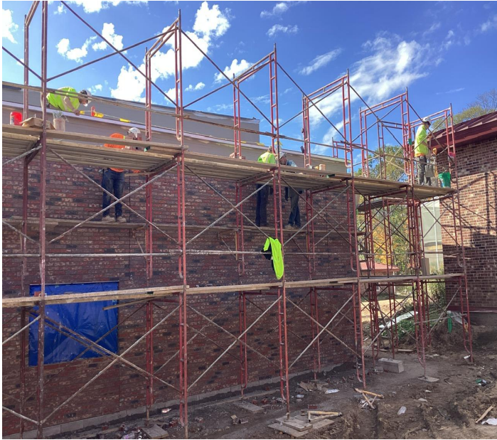
Brick veneer being installed at Media Center addition
