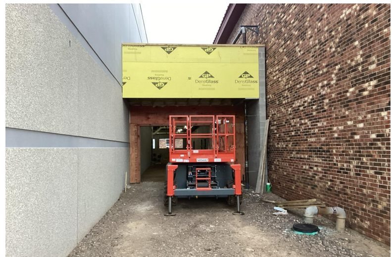
Entrance to gym addition corridor installed
