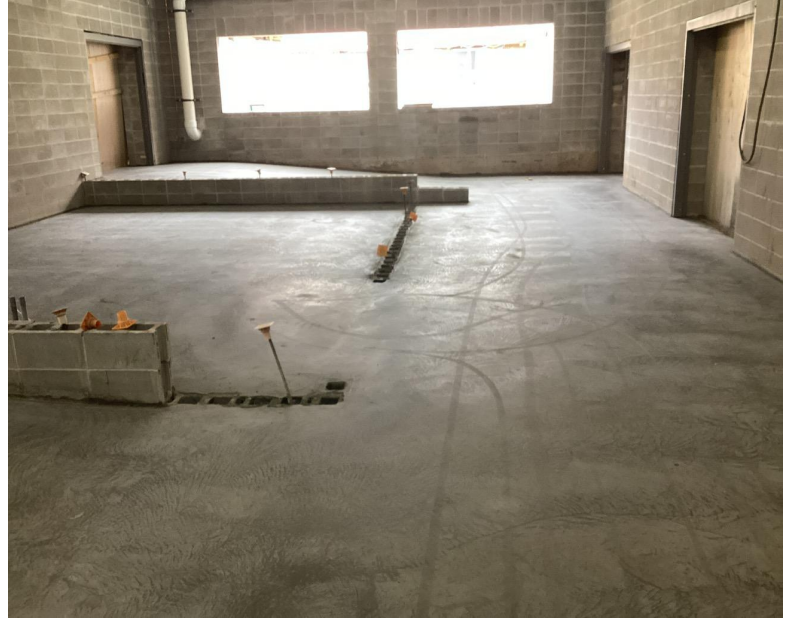
Slab floor poured in Gym addition corridor
