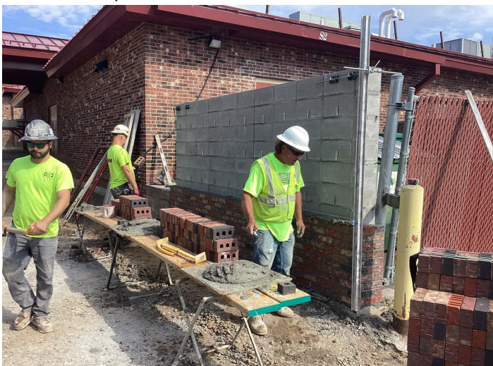
Trash enclosure wall replaced
