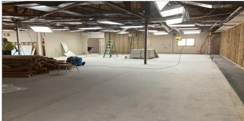
Existing Library Demolition Complete
