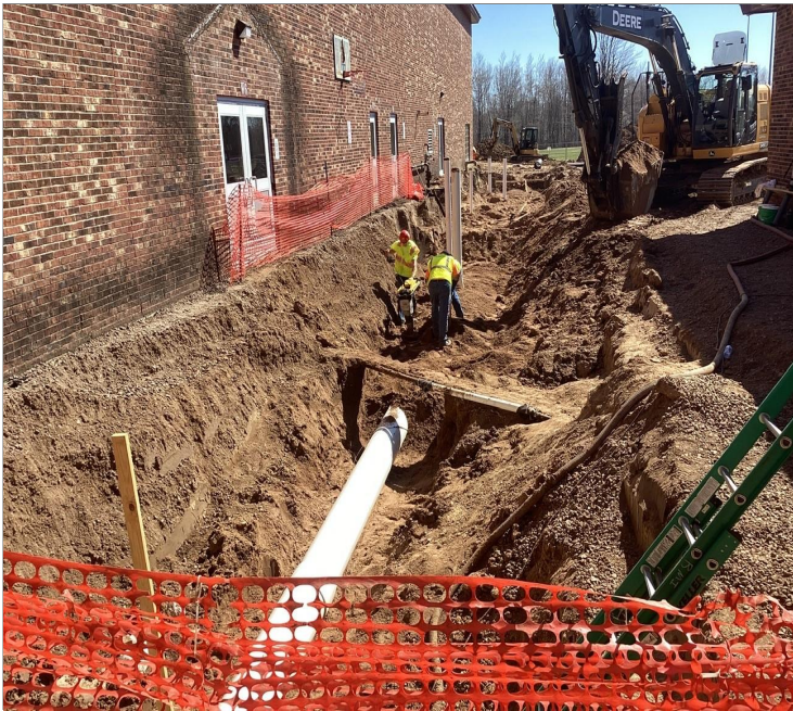
Storm Sewer Installation
