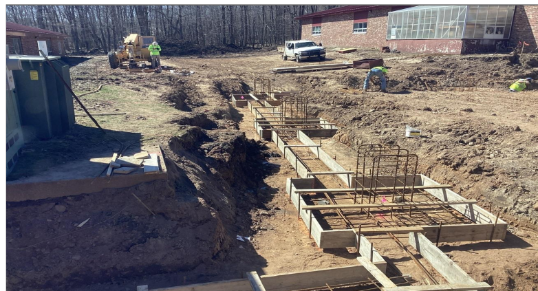
Media Center Footings Formed
