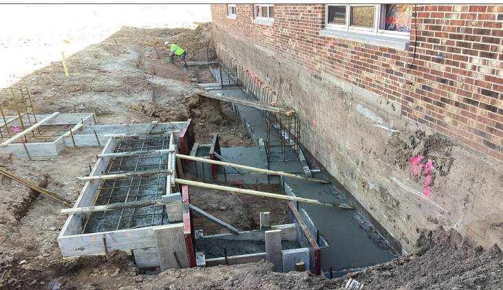
Media Center Footings Poured
