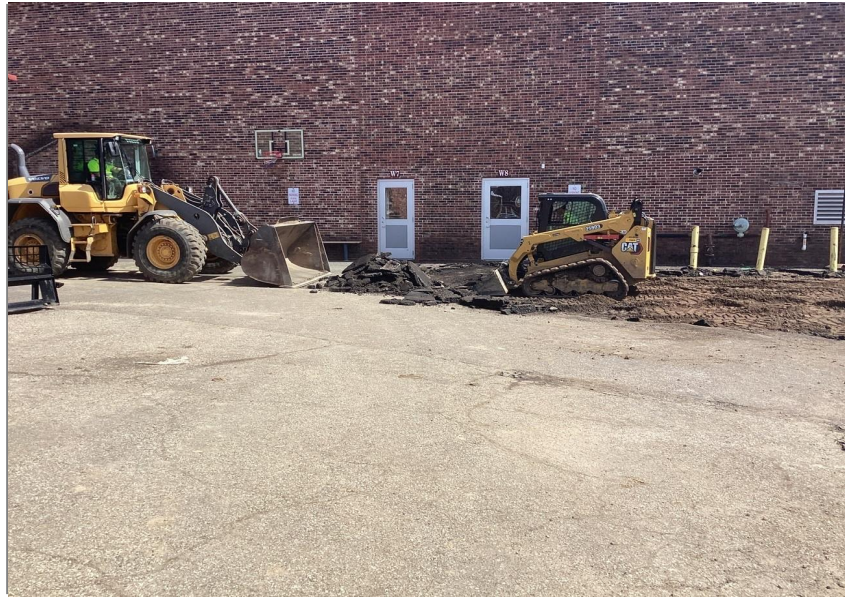
Asphalt Demolition at Gym Addition
