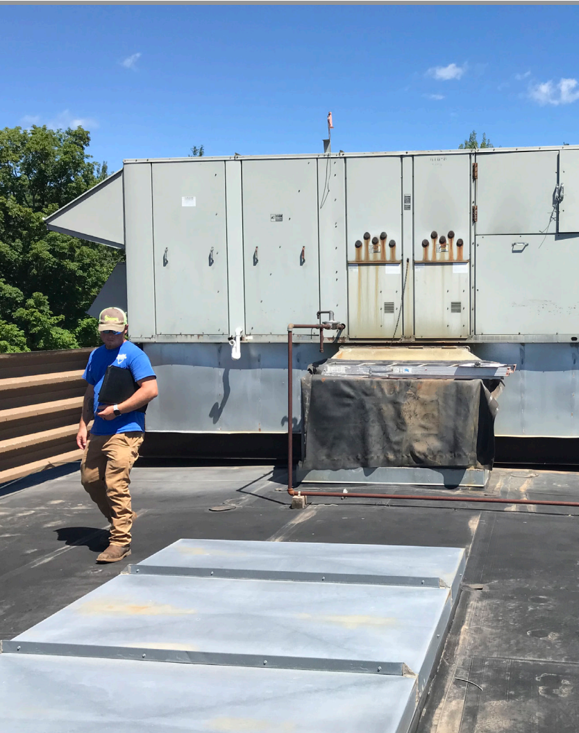
JULY 21 WALK THROUGH AND ASSESSMENT OF THE MS / HS ROOF
